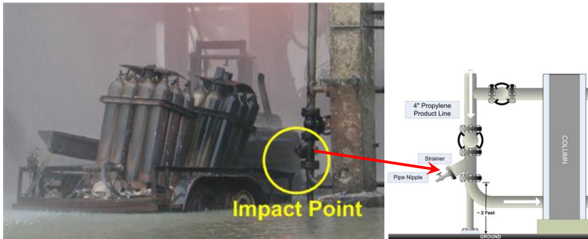
Figure 7 – Impact Point Showing Damaged Y-Strainer
